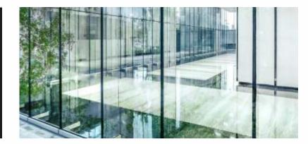
Toughened glass is known for its high mechanical strength and is used in various mechanical fixings. It boasts 4 to 5 times the strength of a regular glass of the same thickness. Toughened glass is also thermal shock resistant, able to withstand temperatures up to 250°C. Its strength, safety, and thermal resistance make it a popular choice for applications such as elevations, doors, partitions, shower enclosures, railings, balconies, canopies, automatic sliding doors, and more.
