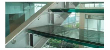
Laminated glass is a type of safety glass made by bonding two or more sheets of glass permanently with a plastic or resin interlayer. The interlayer increases the glass' strength and helps to hold the fragments in case of breakage.
